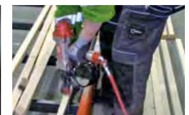
Timber to Metal Stud
