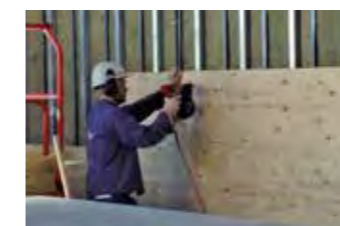
Plywood to Metal Stud
